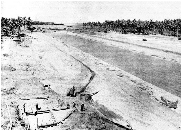
Completed Marston mat airstrip
